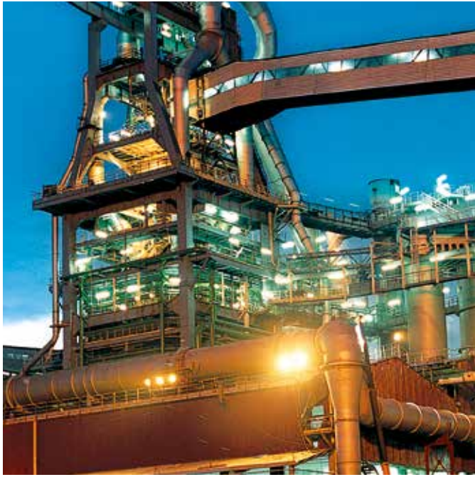
Industrial application: Refinery
