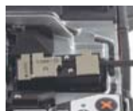
Drop cable splicing with fiber holder system
