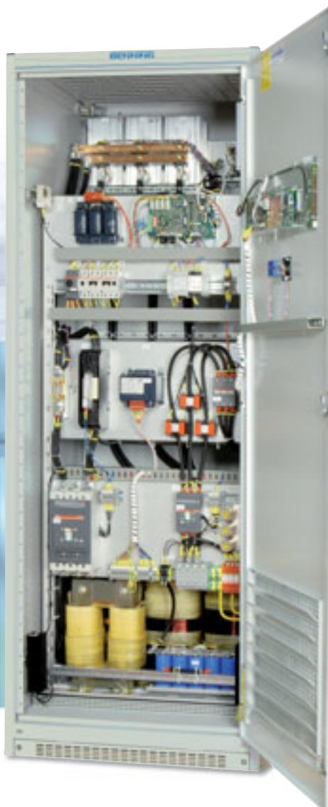
Fig. 4 Thyrotronic interior view
