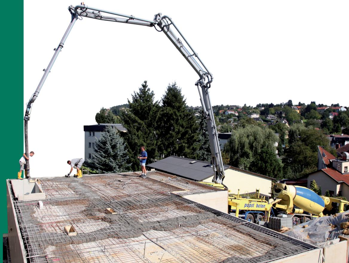
With its lightweight construction, SCHWING is able to achieve a total weight of less than 18 t, without making any compromises in respect to the core pump battery, Rock valve and boom.
